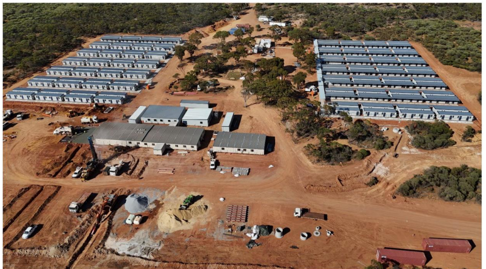
Figure 27 - MGGP camp build nearing completion.
