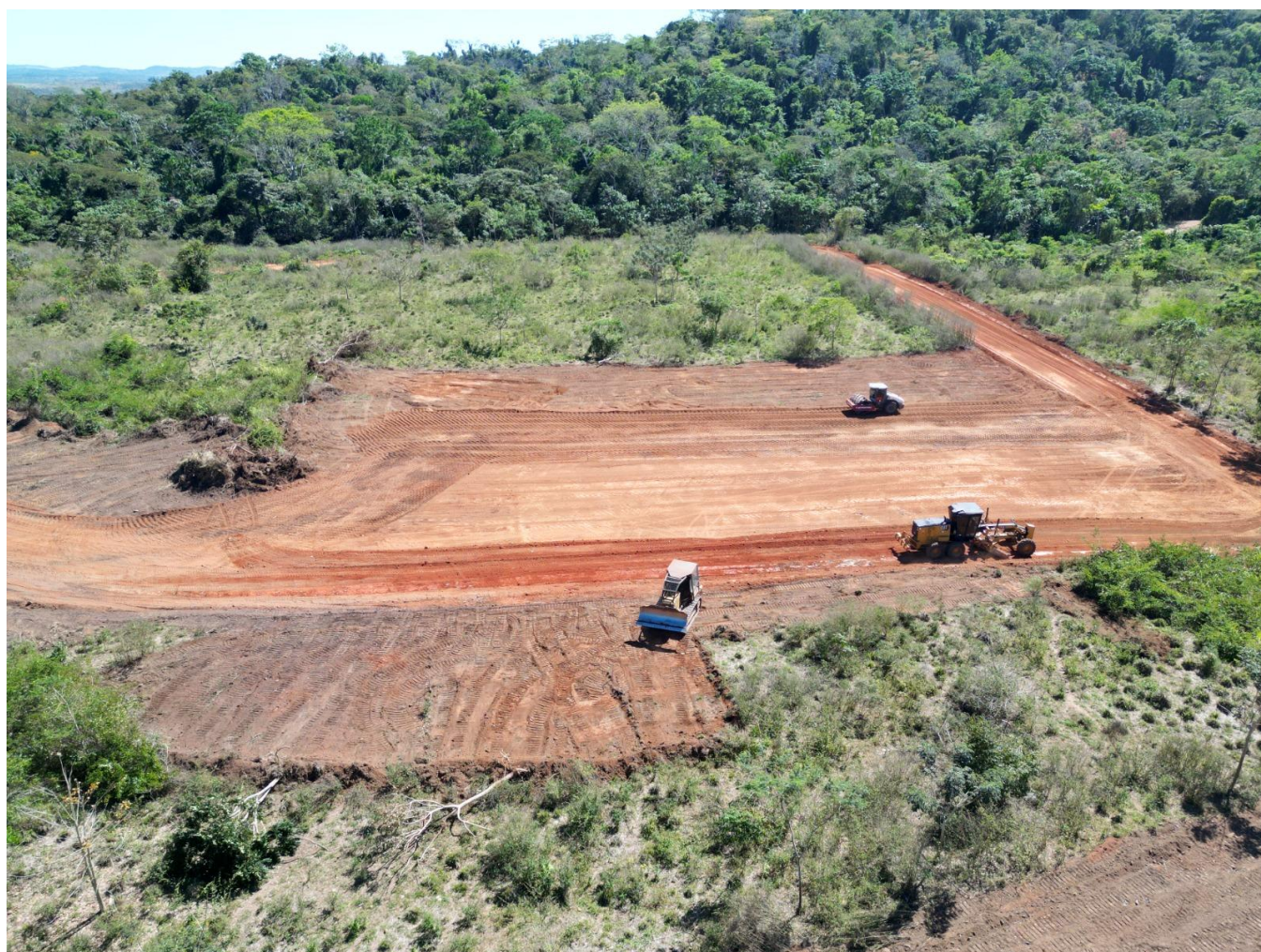
Figure 2 – Jaguar Project Pre-Development Earthworks
