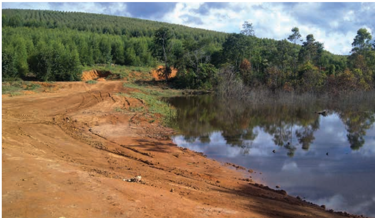
Figure 3 – Completed Temporary Cofferdam
