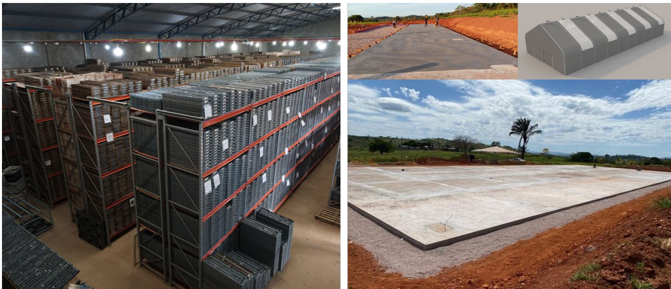
Figure 6 – Existing Core Shed (left) and build of new core shed (right)
