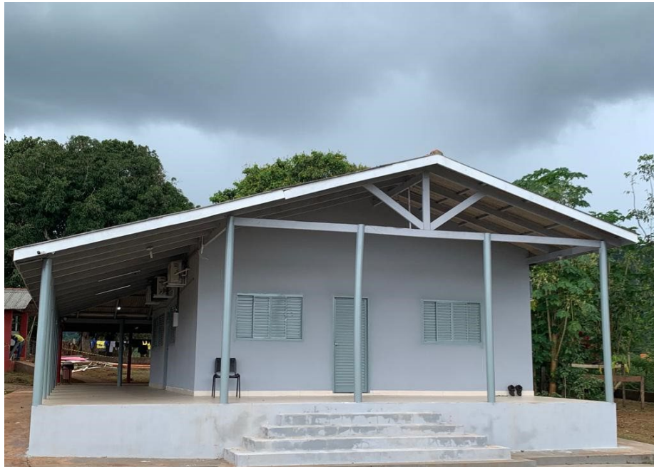
Figure 9 – New On-site Accommodation at Jaguar
