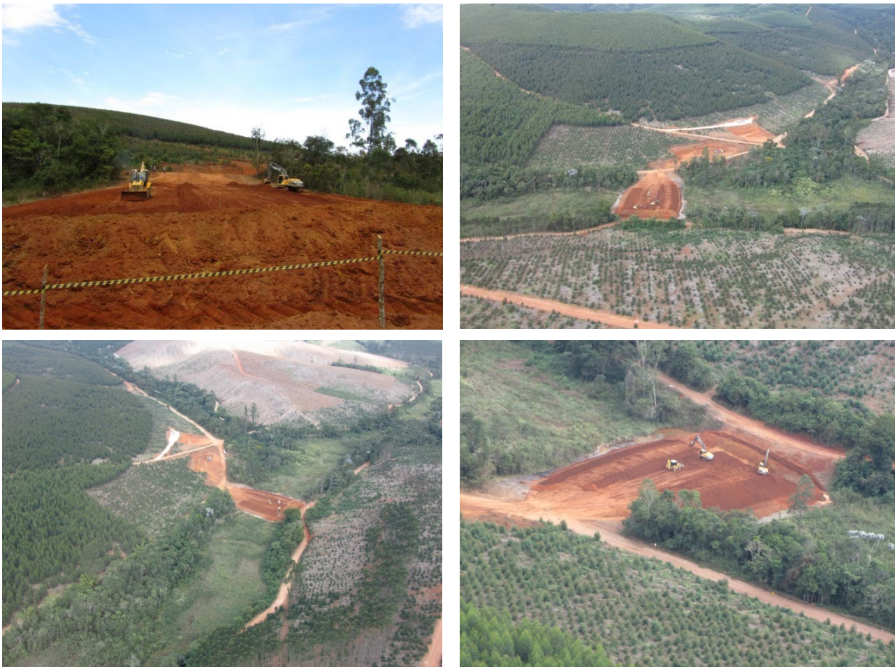
Figure 2 – Temporary Water Dam Construction at Jambreiro
