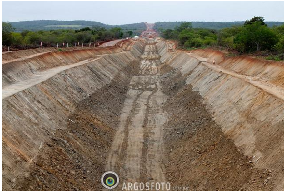
Figure 2 – Transnordestina Railway under Construction in Paraíba State, Brazil
